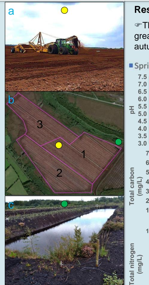
Fig. 1. (a) Peat extraction at an Irish raised bog, (b) aerial view showing 3 catchments, and (c) treatment pond located on the edge of catchment 1.
